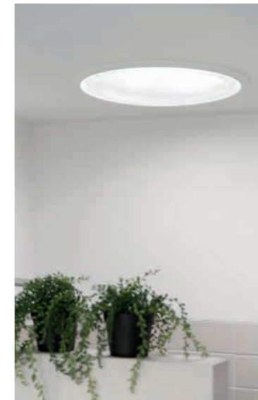
A VELUX sun tunnel leads daylight to the deepest corner of the bathroom in RenovActive.
